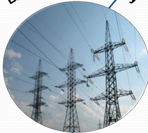
Electrical power supply
