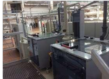
Schmid alkali dip regeneration system (Germany)
