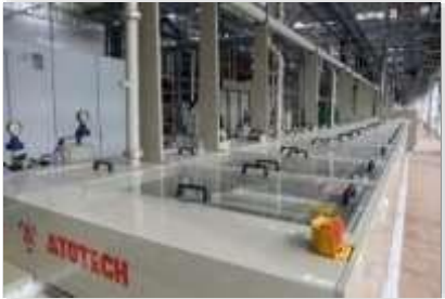
Atotech horizontal chemical galvanic line (Germany)
