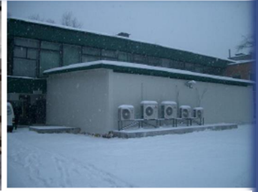
Building for MRI and CT
