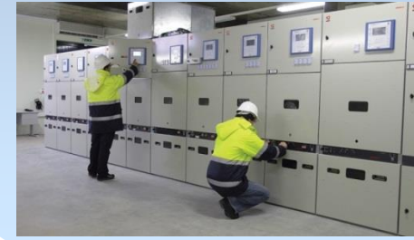
HV & LV DISTRIBUTION GEAR
