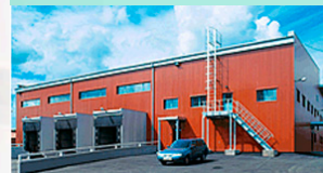
Orion Plastic Pack Factory, Construction Project Sertolovo 2001-2002
