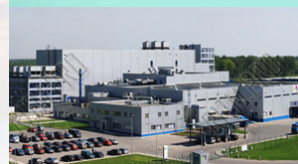
Kraft Foods Factory Reconstruction project 2001-2002
